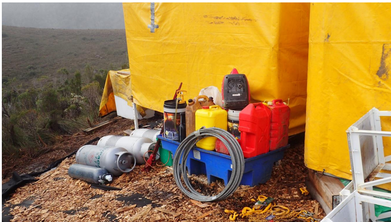
Bund for sundry lubes etc. Note open to weather and required cover to be placed over it (actioned). Note tidy housekeeping.
