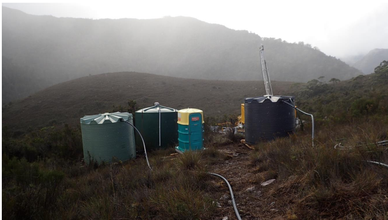
Wet a time of inspection, but water for drilling has been in short supply. Tanks are gravity fed from watercourse with a small catchment. Note the inclusion of an emergency shelter and separate toilet unit.
