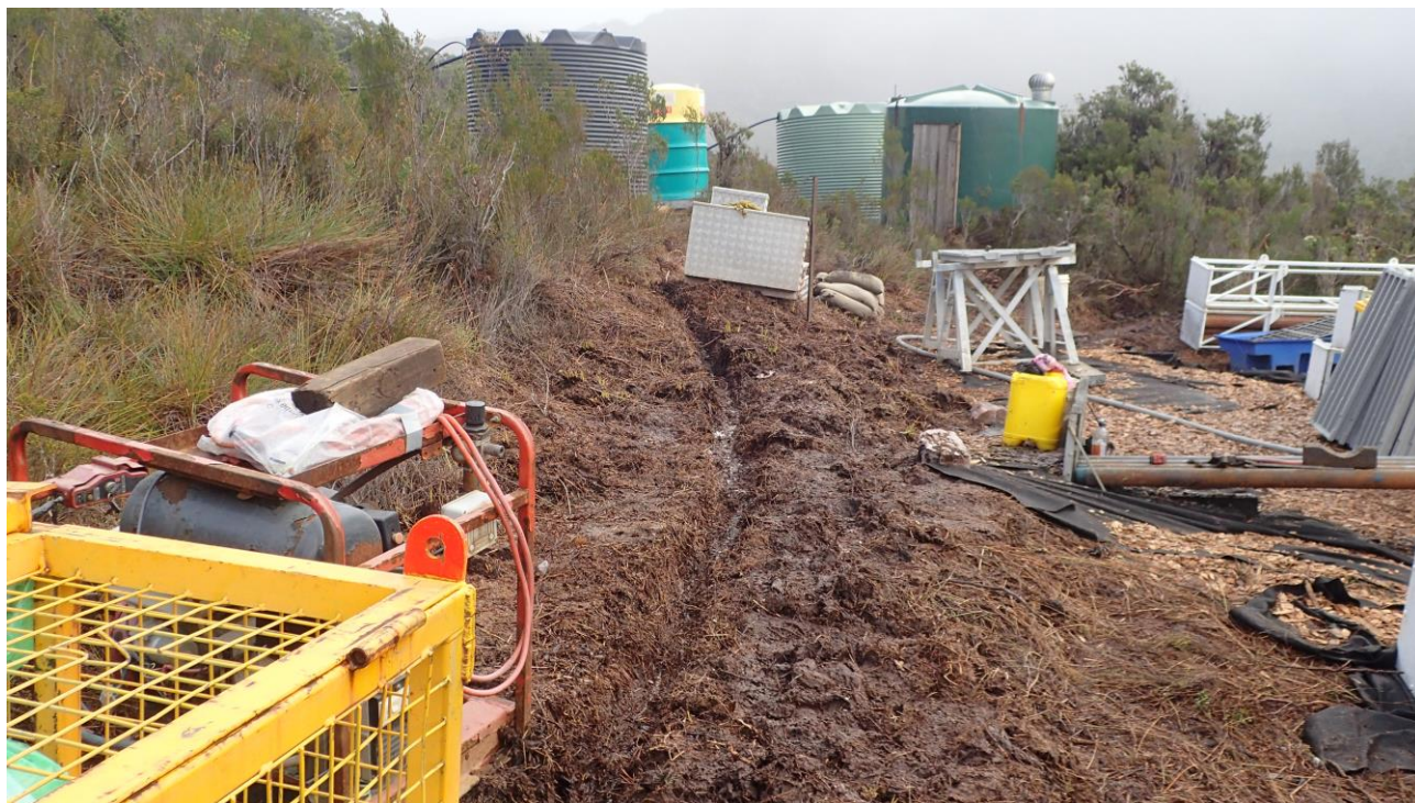
Hand dug trench on the topside of drill pad. Effective in reducing water flowing over the working area (for improved safety and environmental outcomes).
