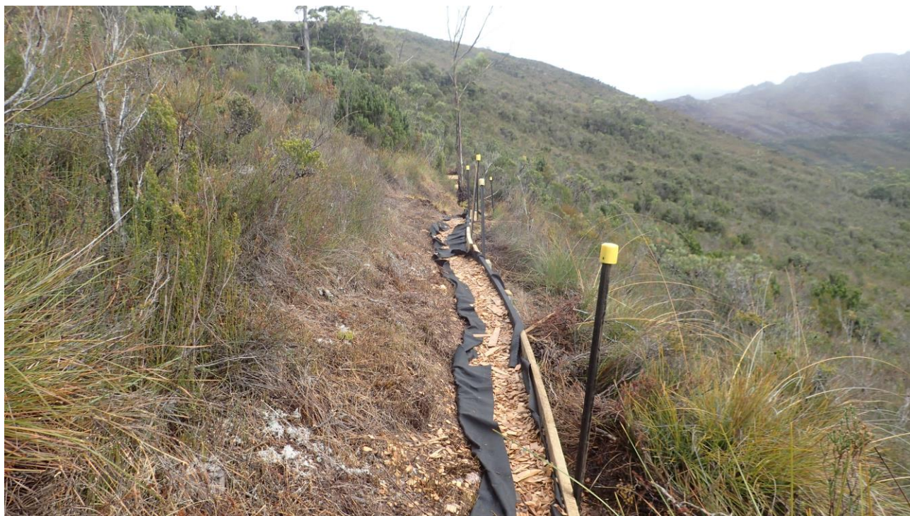
Example of use of treated pine timbers, geotextile mat and woodchips on walking route.
