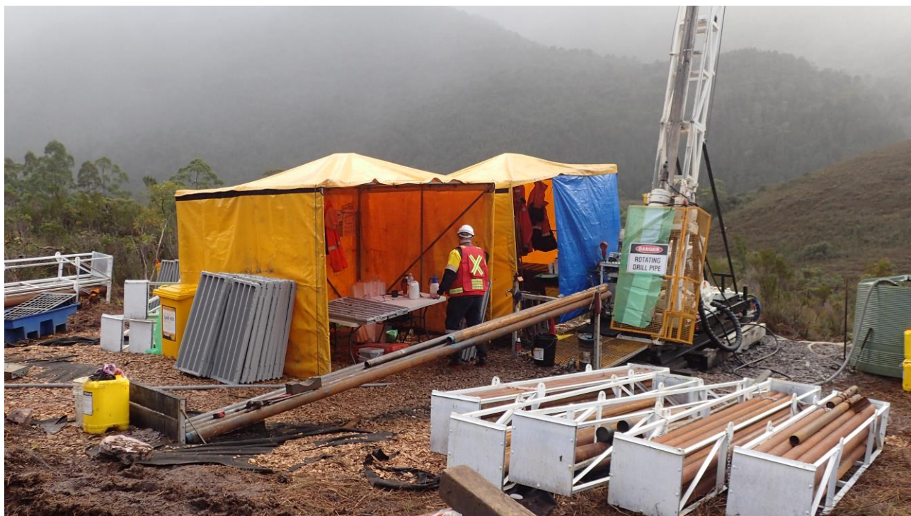
Looking north over section of the site. Note use of heavy duty geotextile and woodchips under the working area.
